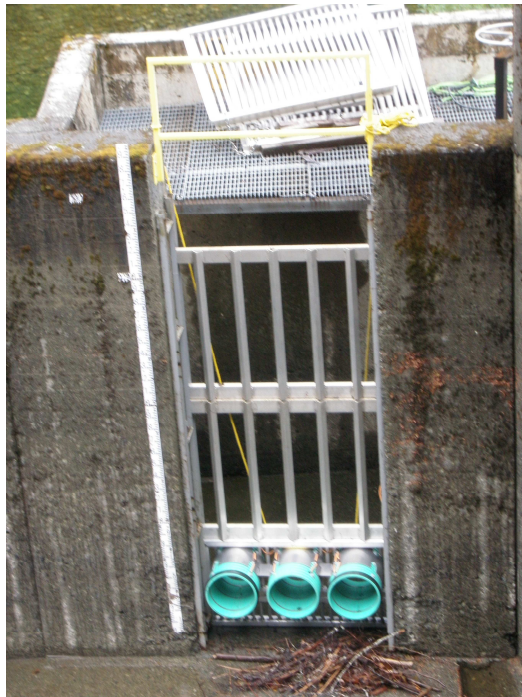
Figure 4. The exit of the fishway with the resistivity counter in place and original trash rack panels in place above counter. The modified trash-rack panels designed to prevent passage of fish above the counter can be seen lying on top of the fishway.
